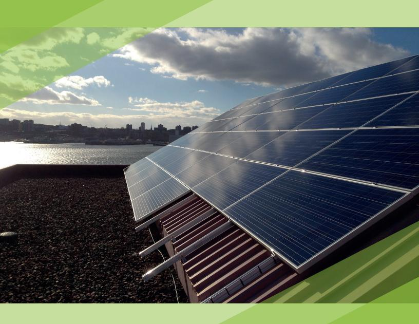
A 12.2 KW COMMERCIAL SOLAR PHOTOVOLTAIC SYSTEM DESIGNED AND INSTALLED BY SOLAR GLOBAL SOLUTIONS FOR THE CITY OF HALIFAX, AS PART OF THEIR CORPORATE EFFORTS TO ADOPT SOLAR AND REDUCE THE CARBON FOOTPRINT OF THEIR FACILITIES
